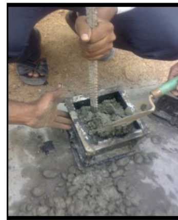
Fig 8- Compaction of concrete
