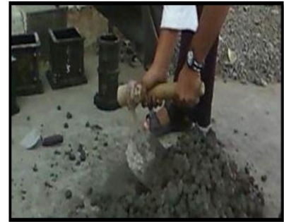
Fig 7- Mixing of concrete
